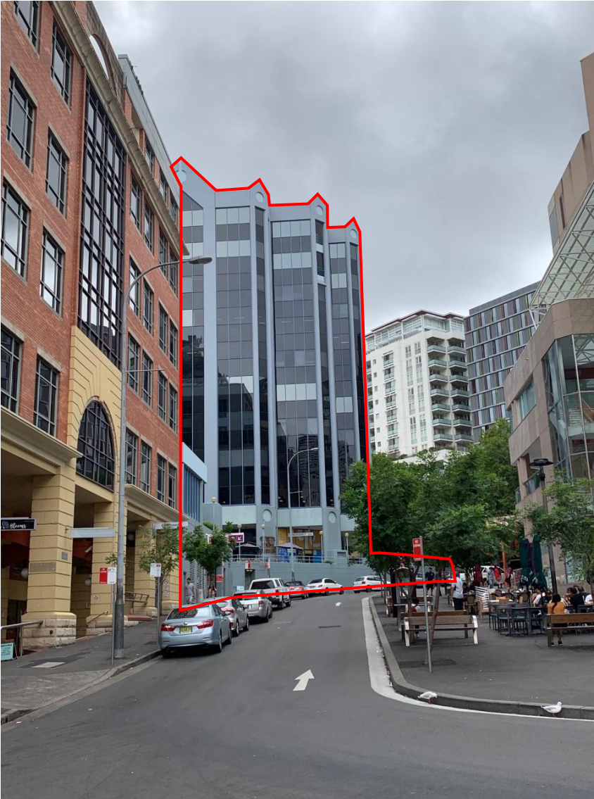
Figure 4. Looking south along Thomas Street towards the subject site, shown in red
